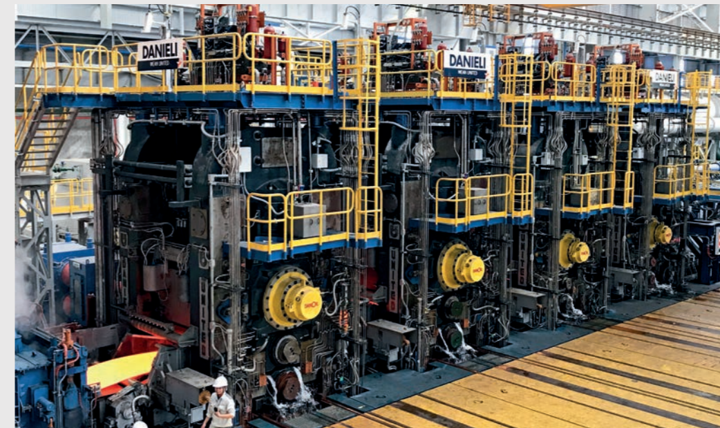
A recent, complete installation of DanOil Bearing at Hoa Phat, Vietnam (Danieli QSP).
