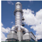
FTP MAIN FANS DRIVE CONTROL
