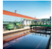
PLANT WATER TREATMENT PLANT
