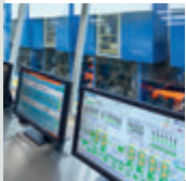
HOT STRIP, PLATE AND COLD MILLS
