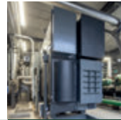
WTP ABSORBER SYSTEM
